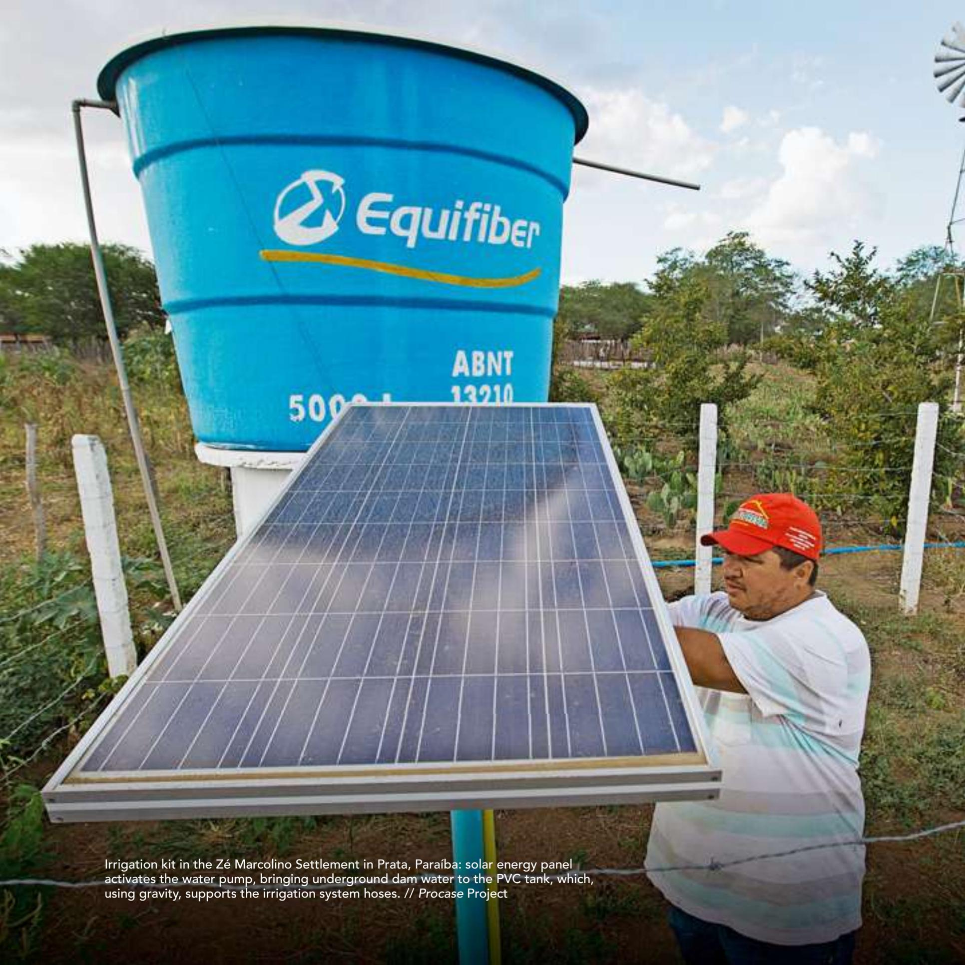
Irrigation kit in the Zé Marcolino Settlement in Prata, Paraíba: solar energy panel activates the water pump, bringing underground dam water to the PVC tank, which, using gravity, supports the irrigation system hoses. // Procasa Project
